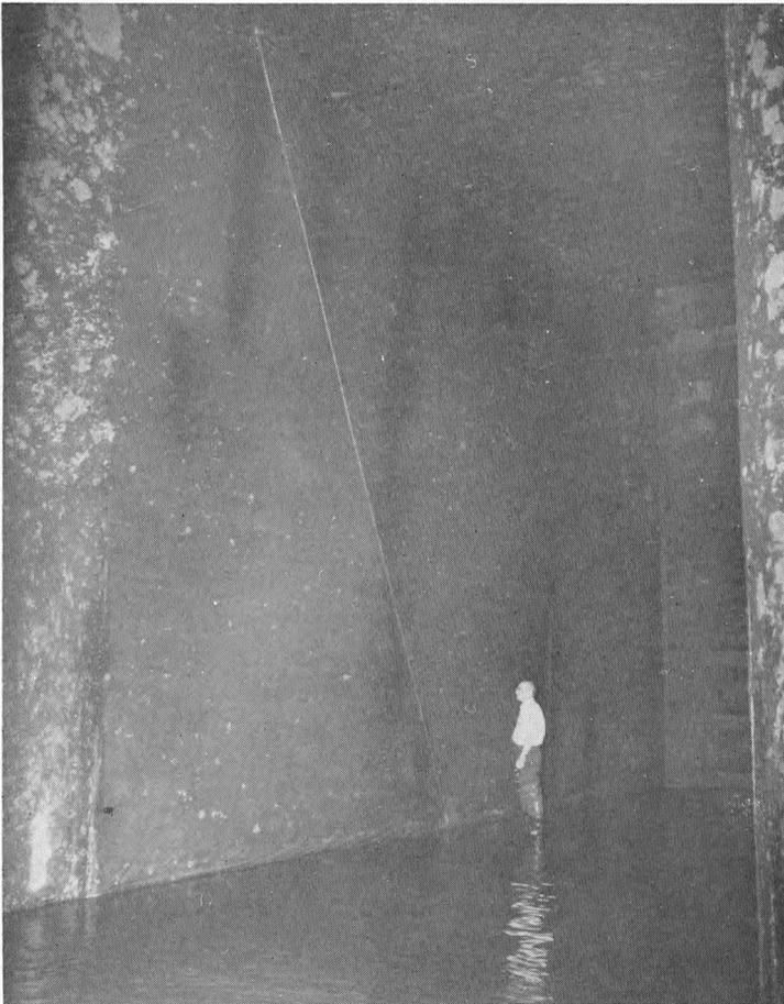
FIG. 6. 30 FOOT TRANSDUCER INSTALLED IN 42,500-HORSEPOWER TURBINE INTAKE
