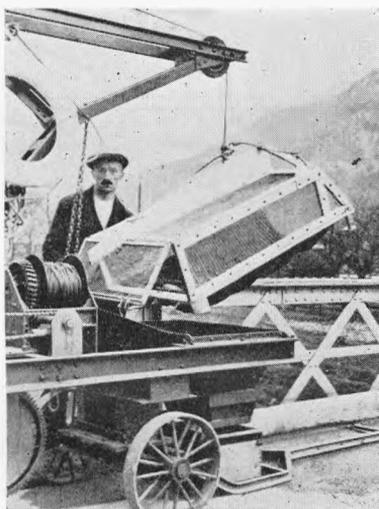
FIG. 1.—BED-LOAD SAMPLER OF THE BASKET TYPE DEVELOPED BY THE SWISS FEDERAL AUTHORITY FOR WATER UTILIZATION.
