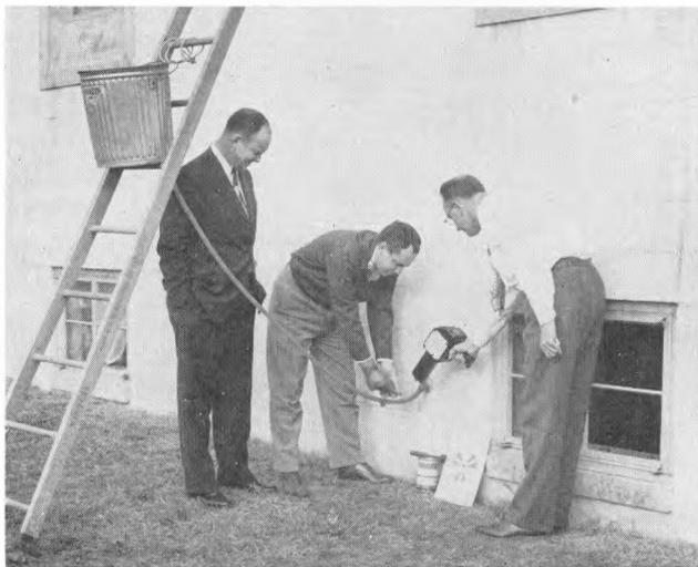
FIG. 11a. TO LOCATE A PUZZLING LEAK BENEATH THE CONCRETE FLOOR IN KERN METHODIST CHURCH, OSCAR BIZZELL INJECTS  $2\frac{1}{2}$  MILLICURIES OF IODINE 131 FROM A LEAD SHIELDED SYRINGE INTO A GARDEN HOSE SERVING AS A PRESSURE HEAD. JAMES HITCH MONITORS THE OPERATION WITH A "CUTIE PIE" WHILE REV. G. WILSON ELLIOTT WATCHES.
