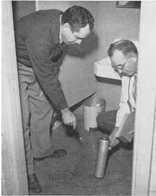
FIG. 11c. AFTER TRACKING THE RADIATION THROUGH SEVERAL ROOMS AND AROUND BENDS IN THE PIPE, THE SIGNAL CAME TO A STOP IN A LAVATORY. A BULL'S EYE ON THE FLOOR INDICATES THE SPOT ABOVE THE LEAK.
