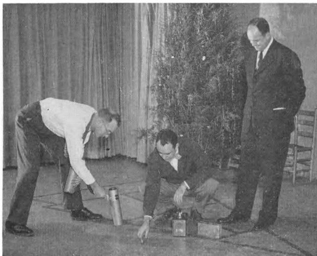
FIG. 11b. HITCH WITH A SCINTILLATION COUNTER AND BIZZELL WITH A GEIGER COUNTER TRACK THE RADIOACTIVE SIGNAL ACROSS THE CONCRETE FLOOR. THE MORE SENSITIVE SCINTILLATION COUNTER WAS FOUND TO BE BEST SUITED FOR THIS TYPE OF MEASUREMENT.
