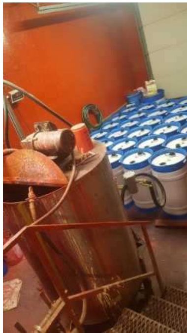
Figure 9. Chemical Storage Room: Excess chemicals are stored in climate controlled and sealed off room
